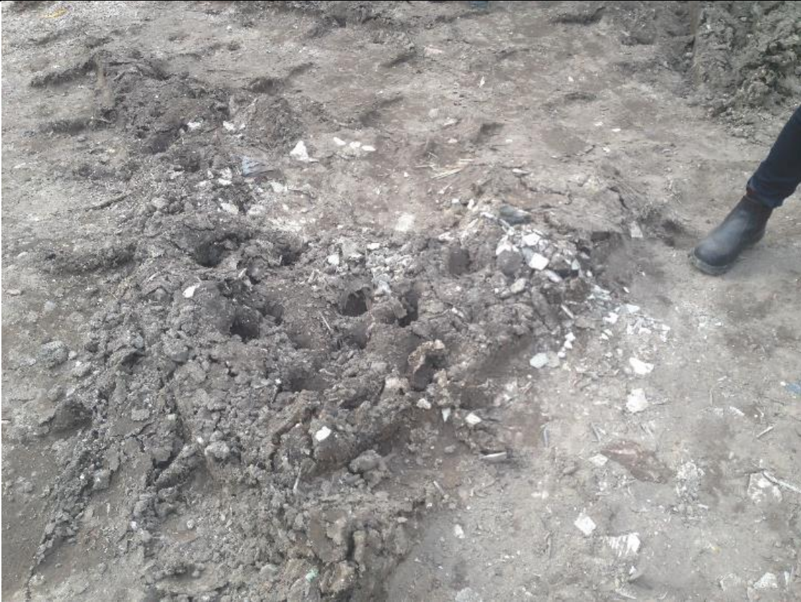
Photograph 1: An overview of the asbestos that was not adequately covered in the Asbestos Disposal Area. Note: Broken Asbestos fragments on the surface and evidence a compactor had driven over the area.
