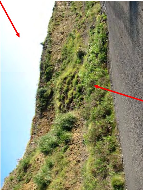
Landslip within shale/soil slope
