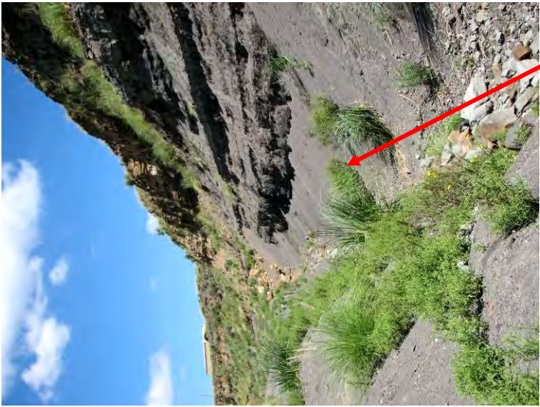
Debris collecting in berm
