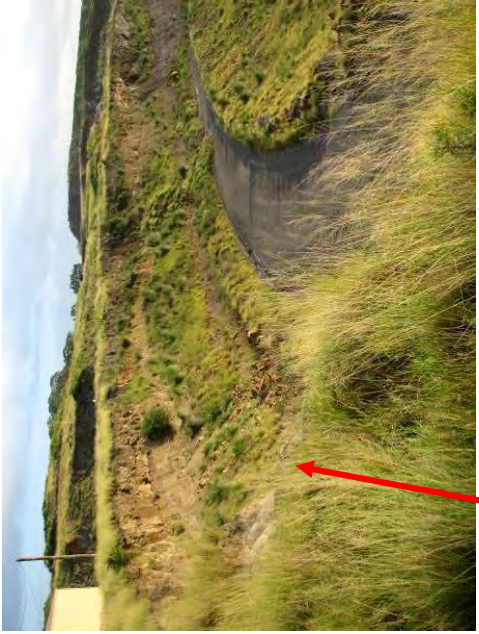
Shale slope with sandstone cap
