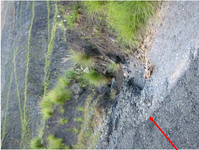
Erosion of crest safety bund
