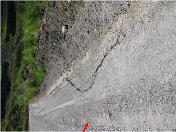
Tension crack in Haul Road above landslip
