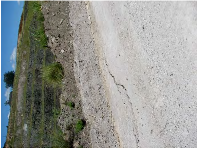
Tension crack in Haul Road above landslip
