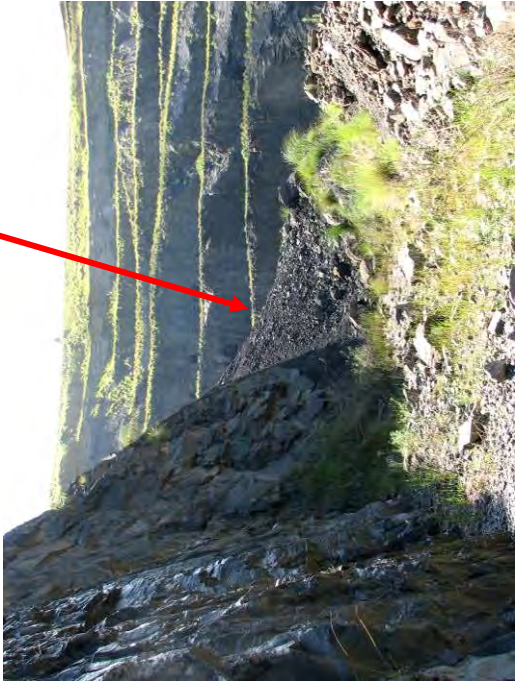
Debris collecting on berm (see Figure 4)
