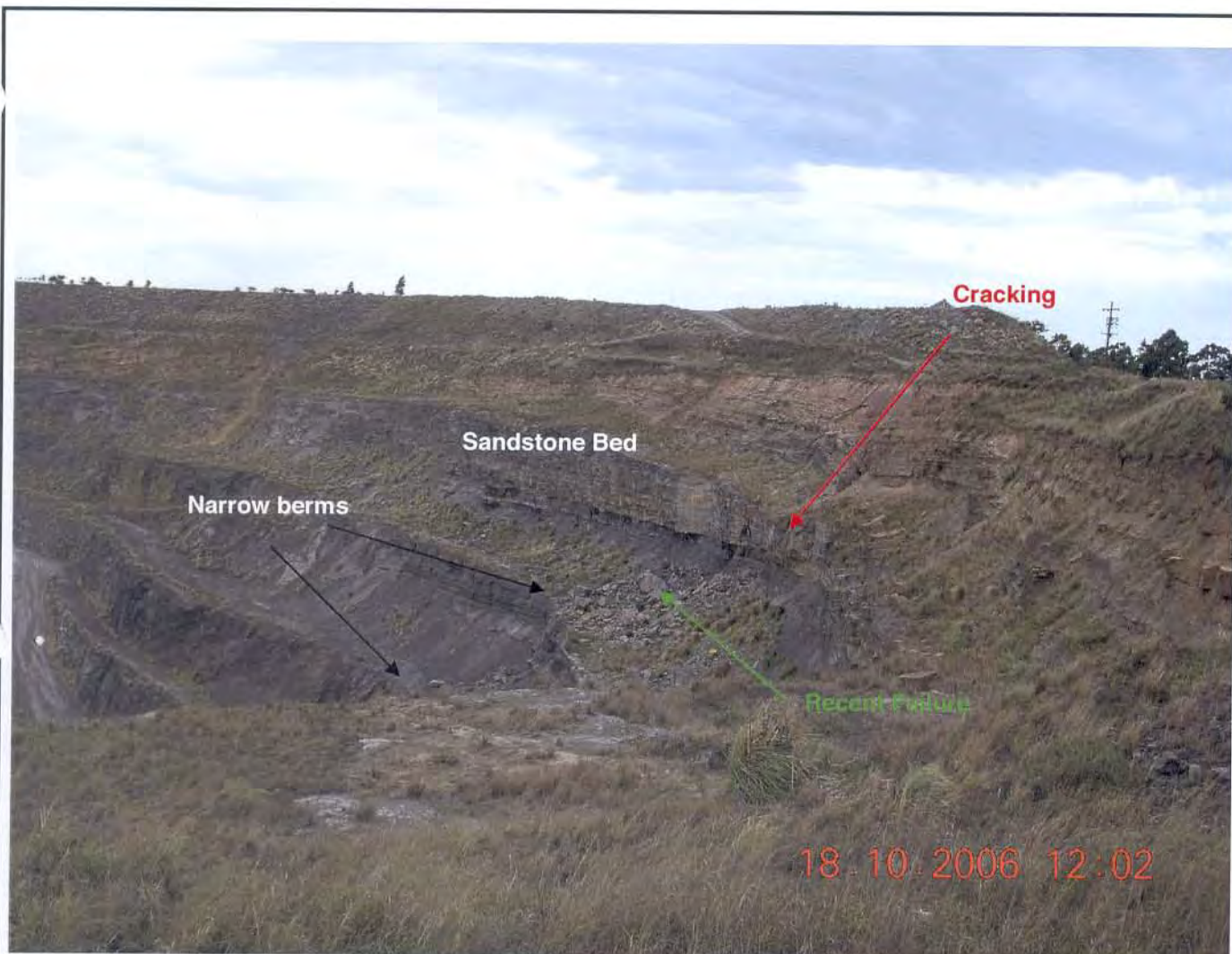
Plate 7 : West wall looking to the north, highlighting undercutting of sandstone bed, narrow berms below, recent failure and cracks within sandstone bed.
