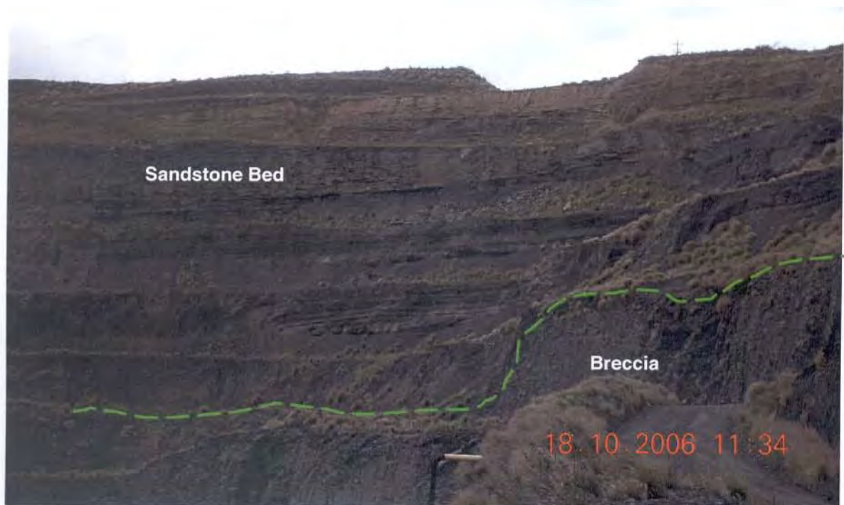
Plate 9 : Overview of upper west wall, highlighting sediments and undercutting of sandstone bed in the area.
