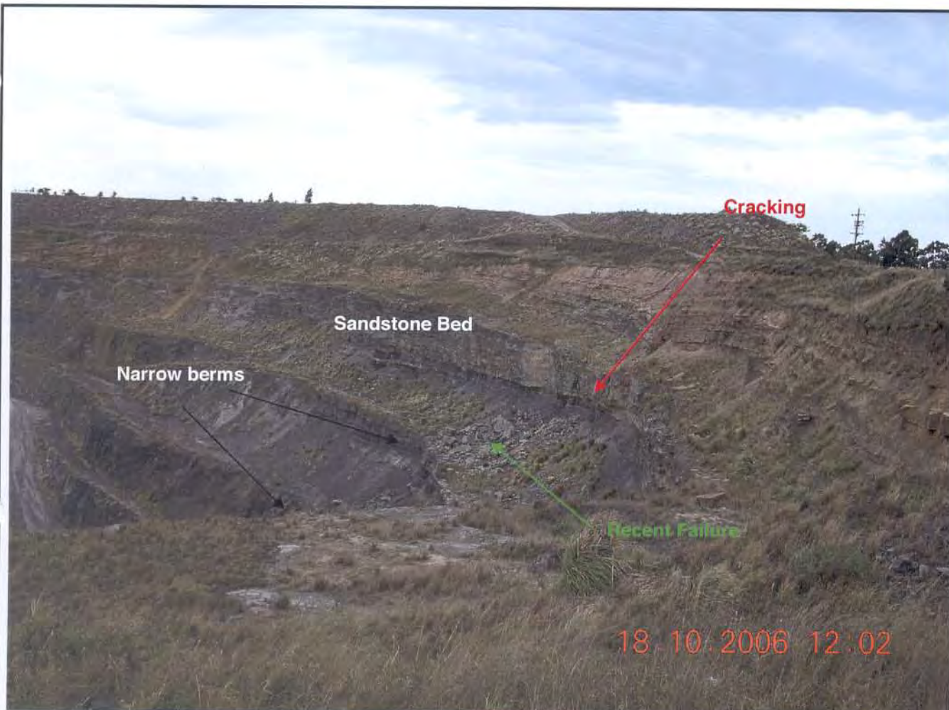
Plate 11: West wall looking to the north, highlighting undercutting of sandstone bed. In long term sandstone ledge will continue to be undercut and with further block fall out anticipated. Process will arrest once a continuous rill slope is formed. Potential for cracking and encroachment behind existing crest.
