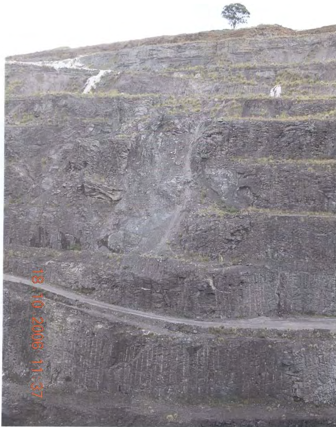
Plate 3 : North wall, highlighting area of instability which initially failed in 2001. Potential for blocks to fall onto road exists. Ongoing monitoring of area required.
