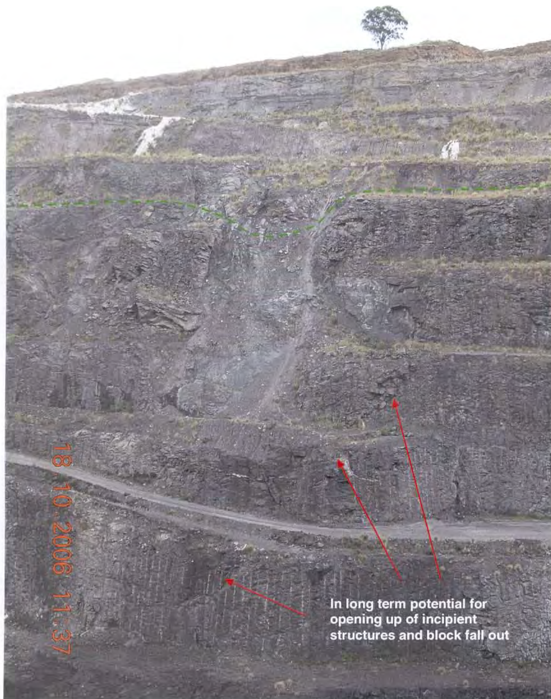
Plate 5: North wall, highlighting area of instability which initially failed in 2001. In the long term, opening up of incipient structures can be anticipated. Furthermore, existing rill will continue to gravitate downwards.
