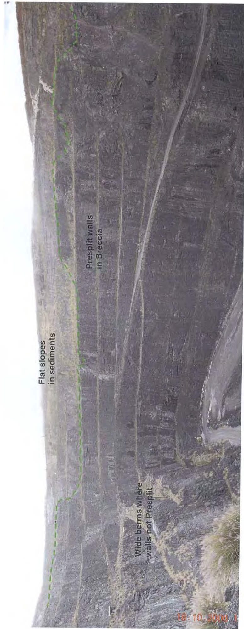
Plate 1 : Overview of west wall, highlighting predominantly pre-split walls within breccia. Generally flat slopes have been developed in the overlying sediments. In the long term rock falls can be anticipated owing to ongoing degradation of breccia. Highest risk is in upper most bench in the breccia near the contact with sediments.
