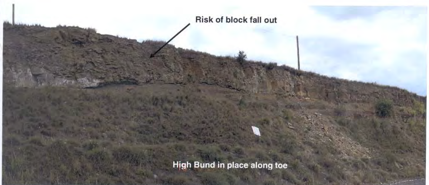
Plate 2 : Upper west wall, highlighting undercutting of sandstone bed with potential for block fall out. Road below is at low risk owing to bund in place. However there is a risk to road immediately above.
