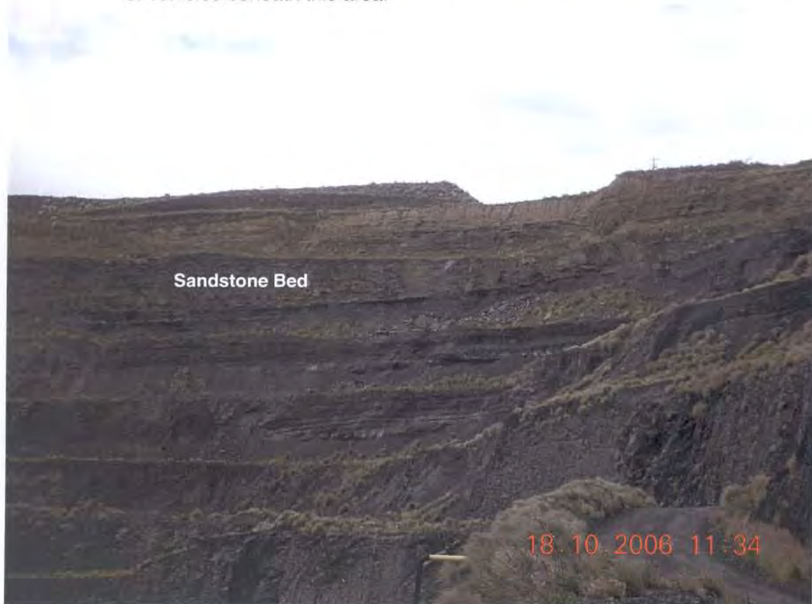
Plate 6 : Overview of upper west wall, highlighting sediments and undercutting of sandstone bed in the area.
