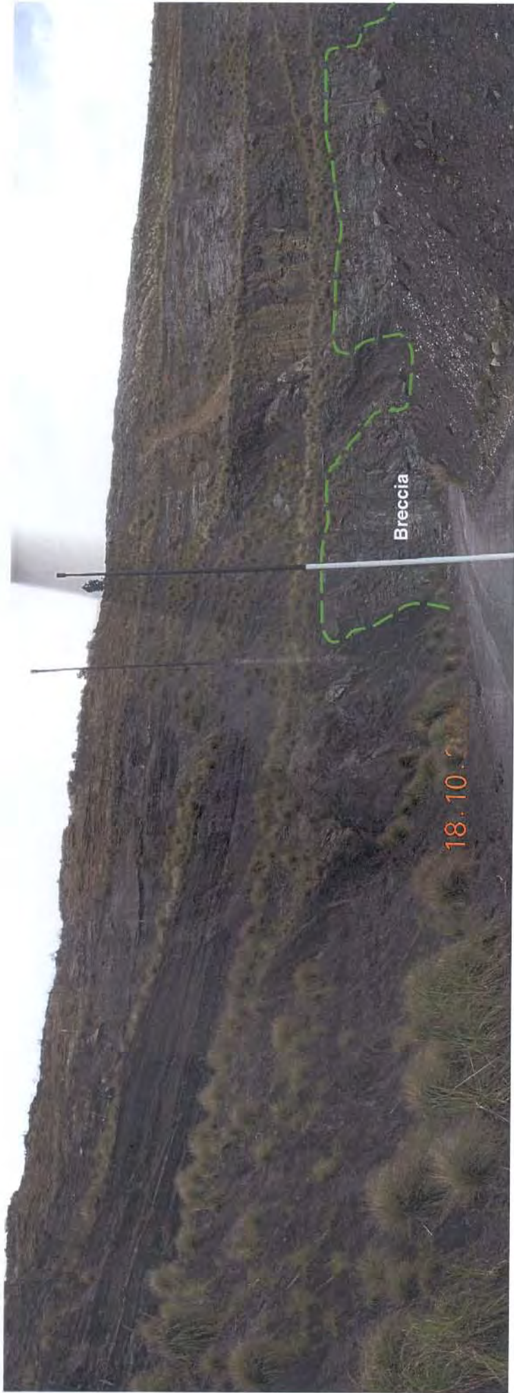
Plate 8: North east quadrant of quarry. Note large rill slopes developed, above breccia. In long term an overall rill slope will be developed.
