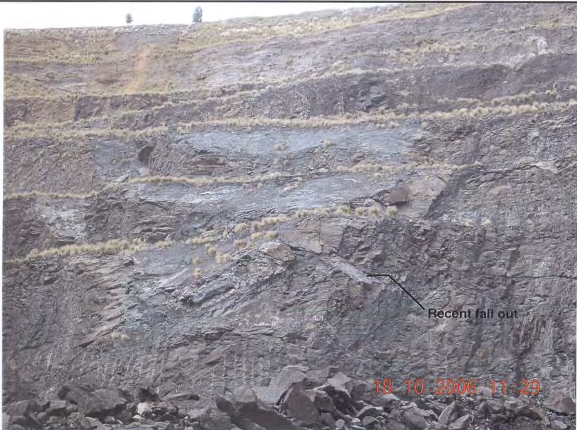
Plate 5 : West wall immediately above haulroad, highlighting area of recent block fall out. All operations personnel need to be made aware of no standing/parking of vehicles beneath this area.
