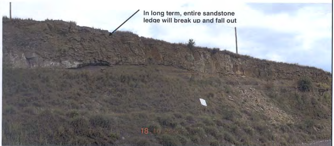
Plate 4: Upper west wall further south of Plate 3. In long term sandstone ledge will break up and fall out. Road above and power poles may need to be relocated.
