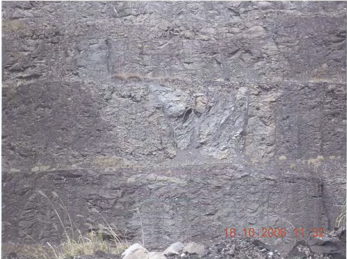
Plate 2: Small areas of walls within breccia, particularly in upper most benches, have entrapped sediments or are very close to sediment contact. These areas are more prone to block fall out.
