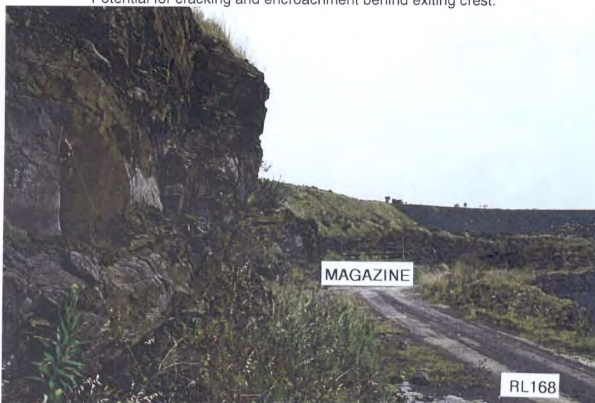
Plate 12: Upper most north wall. Toppling block pointed out as issue in PSM497.R1. Block can either be pulled down or the road closed off.
