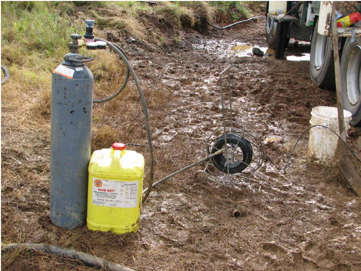
Compressed air source to inflate the packer down hole – packer inflation hose is visible on the reel
