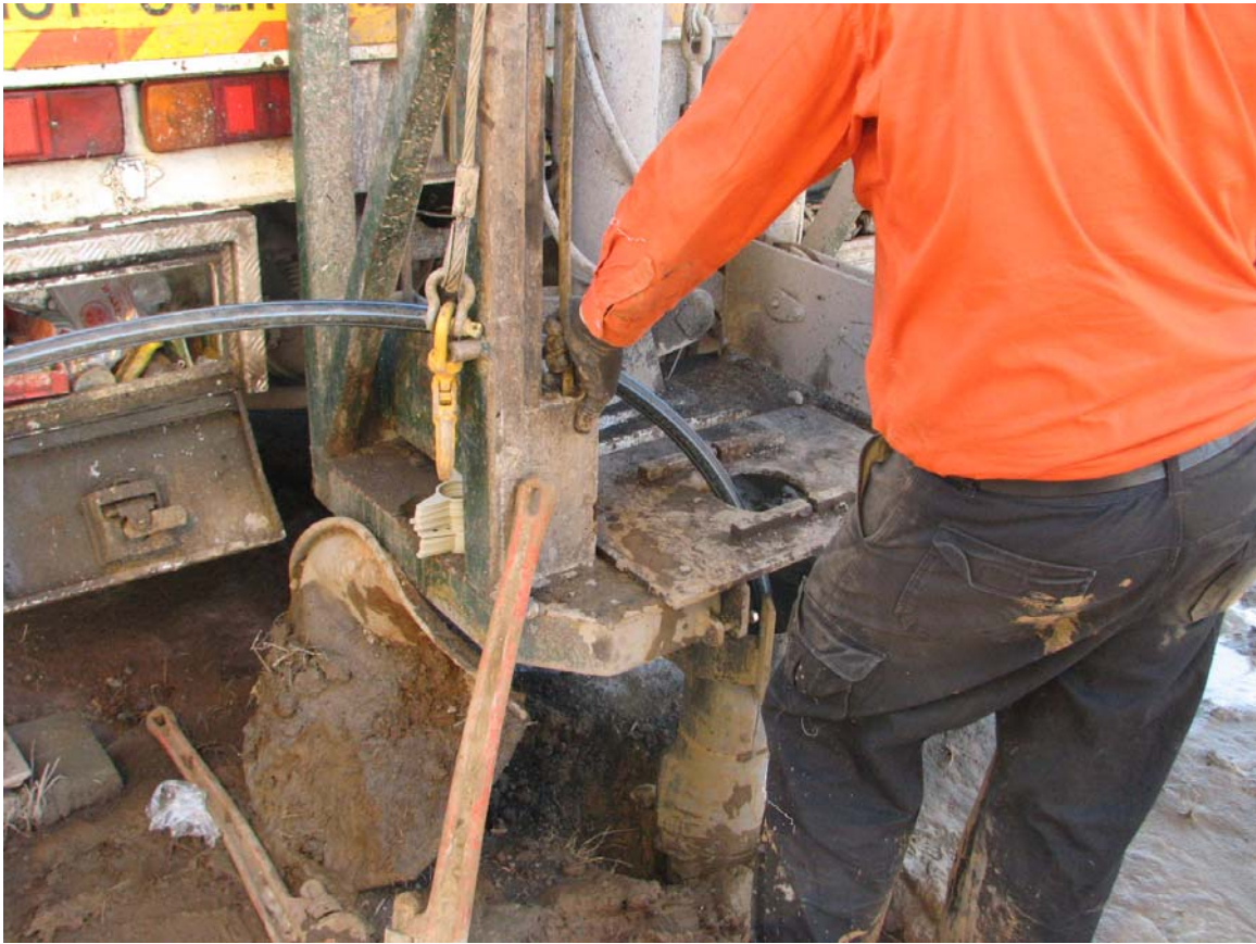
Clean municipal supply water was used to fill drill holes prior to installation of piezometers.
