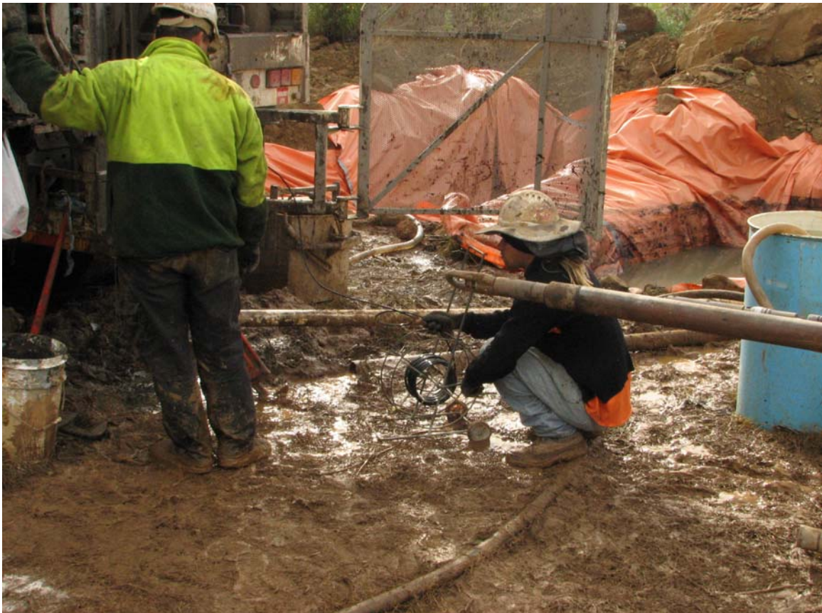
Feeding packer air hose down hole with the packer assembly. The air hose is taped to the cable suspending the packer.
