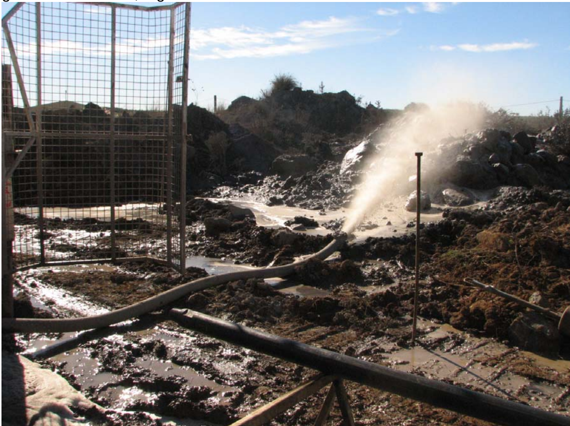
Holes were flushed with water and with biodegradable foam, to remove remaining cuttings, prior to filling holes with water and installing the piezometers
