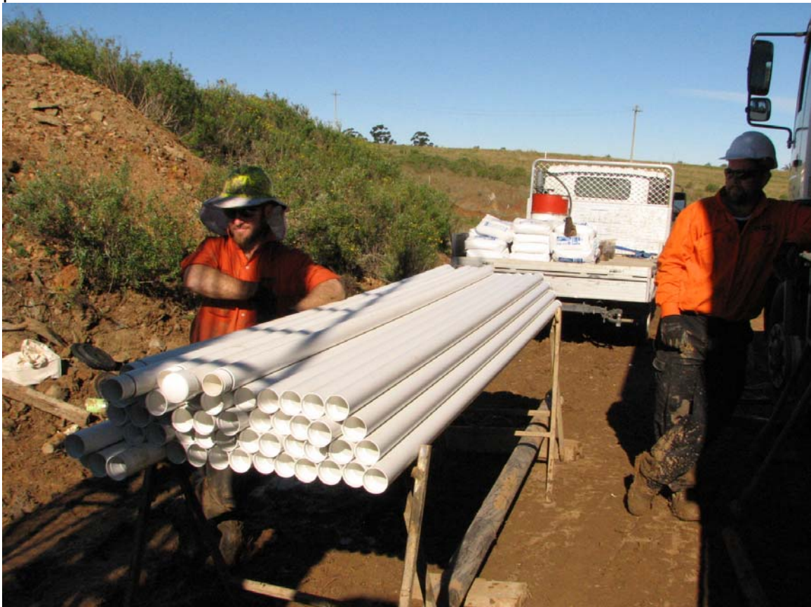
Piezometer materials for installation. Class 19 screwed PVC was used, with plastic centralisers used every 9 to 12 metres to keep pipe central in the hole. A lifting sub was used to lower pipe into the hole.
