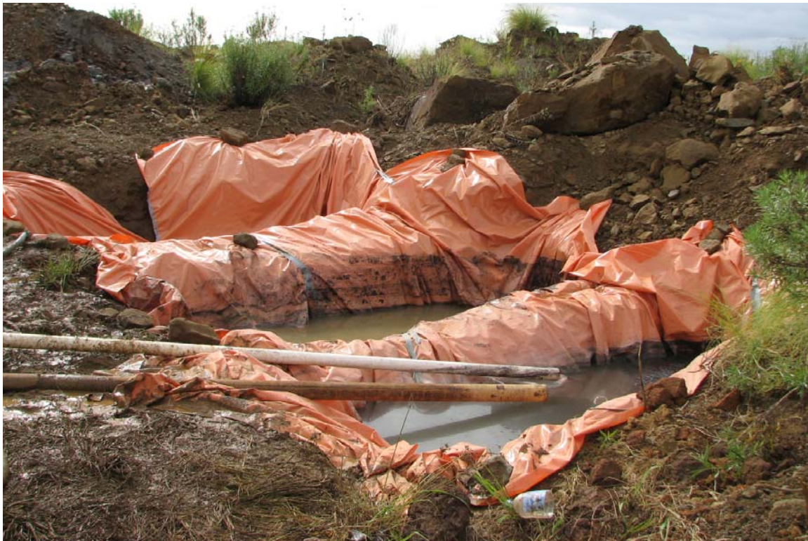
Flushing dirty water with cuttings into pits prior to packer testing
