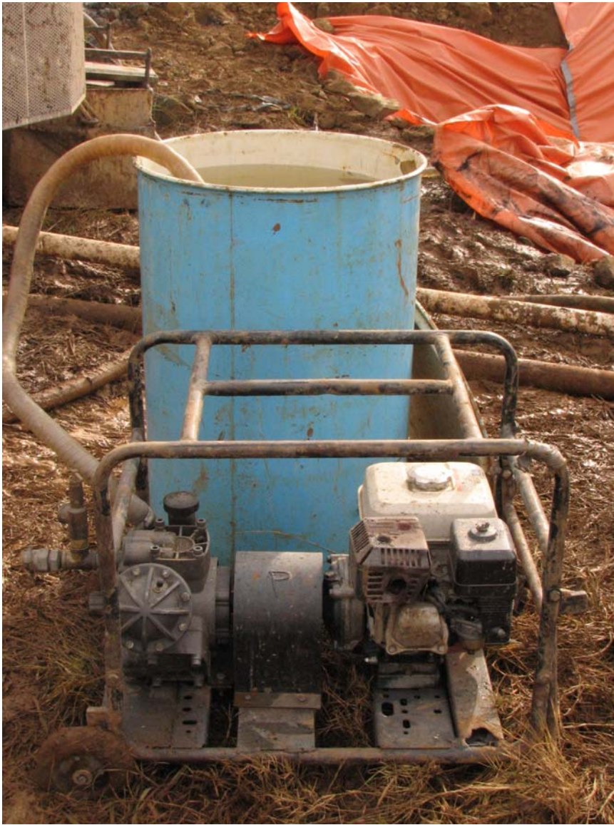
The pump and drum used to hold clean water for packer testing, after the hole has been flushed with water from pits to remove silt that might prevent sealing of the packer.
